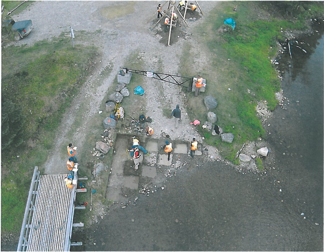
Figure 1 - Aerial view of excavations nearing completion at Bathurst Lake North on August 18, 2016.
