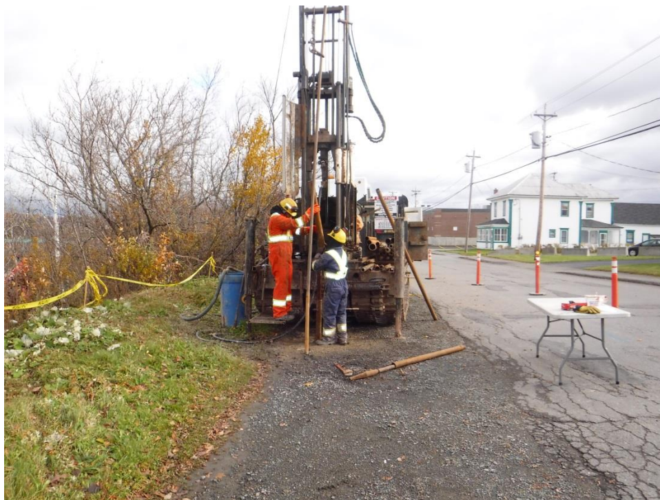
Above: the GHD coring crew working on Front Street.
